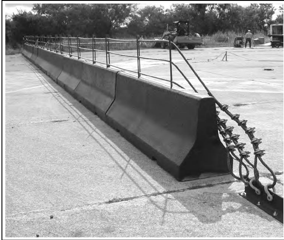
Figure 4-3. Jersey barriers connected with a cabling and anchor system
