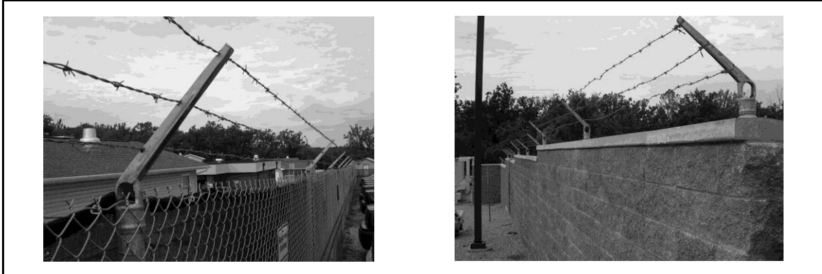
Figure 4-8. Single top guard barbed tape
