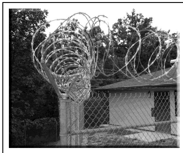
Figure 4-10. Double top guard enhanced with concertina or barbed tape
